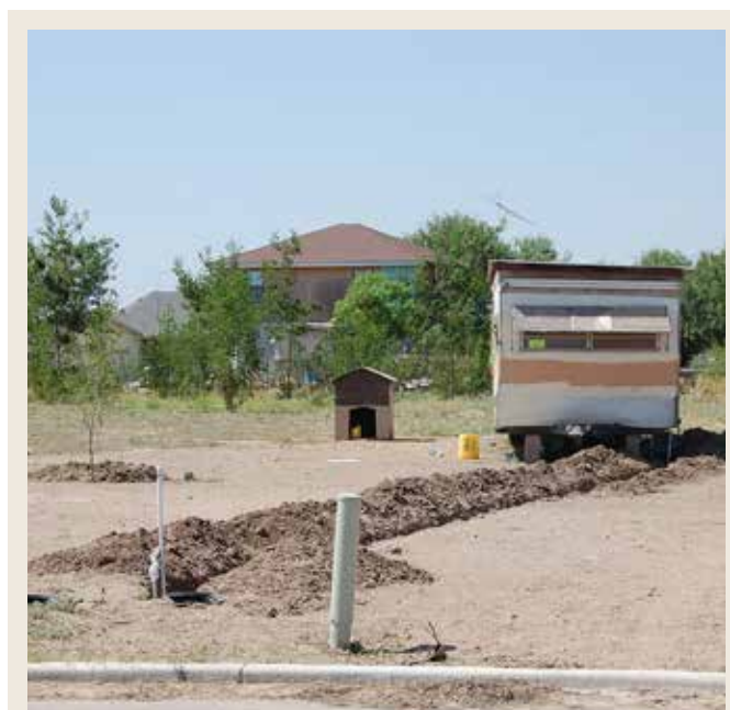
The owner of this RV, located in a legal subdivision in Hidalgo County, has built a small pipeline connecting the home to the subdivision's water line. This subdivision has access to water, sewer, electricity and paved roads. Photo credit: Federal Reserve Bank of Dallas
