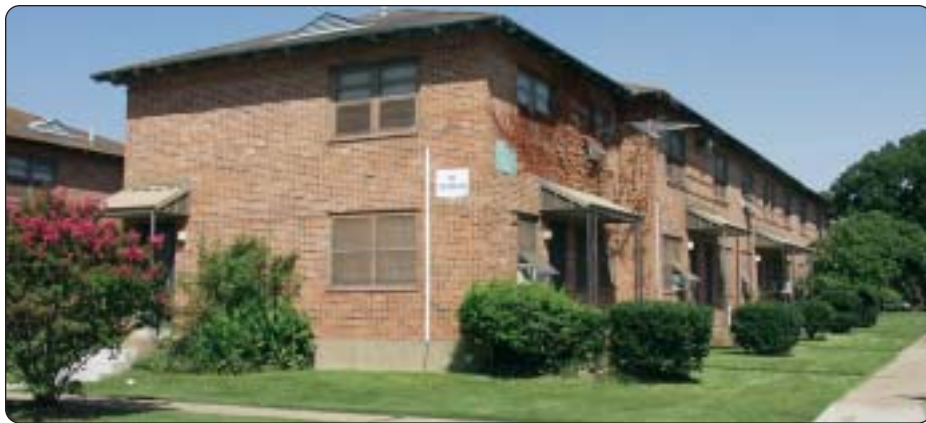
Roseland Homes, a Dallas public housing project, was built in 1942.
