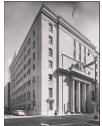
Federal Reserve Bank of Dallas, 400 S. Akard St.
